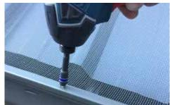
**STEP 3.** Place the standard or Mesh Lock trim over the mesh. The mesh should rest under and against the front edge of the trim. Secure by placing a metal screw in every pre-made hole. If trim is not used, screw the mesh to the gutter edge every 250mm.
