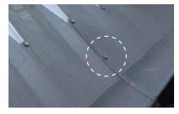
**STEP 5.** Tie the gutter mesh sheets together at the overlaps using a metal screw. One screw per overlap evenly spaced is sufficient.
