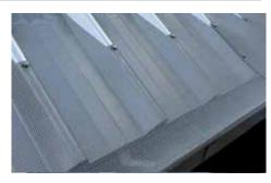
STEP 6. Ensure you've attached the mesh to the roof at all the ridges
