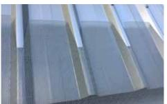
**STEP 2.** Fit the formed edge of the gutter mesh onto the outer edge of the gutter and lay the top edge onto the roof, making sure that the "U's" are aligned correctly with the ribs of the roof sheet. Depending on your gutter type, you may need to pinch the formed edge of the mesh to achieve more of an overlap onto the gutter lip.
