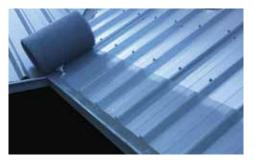
STEP 2. Roll the mesh out along the gutter edge.
