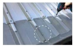
**JOINING MESH** When joining two pieces of mesh, overlap the mesh by 20mm. Place one metal screw through the centre of the overlap.
