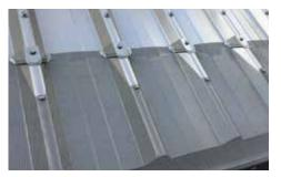
**STEP 7.** Install one saddle on each of the ribs in the roof sheet to hold the mesh against the pan. 2mm back from the leading edge is normal. Attach using a metal screw.
