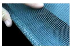
**STEP 1.** Place the roll of mesh on the roof. The edge of the mesh should rest on top – and just inside – the gutter edge.
