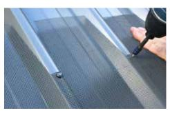
**STEP 3.** Push the mesh toward the gutter and hold with slight tension against it, then place a metal screw through the mesh into the roof on the ridges at the bottom of the "U"s to hold the mesh in place. Do not over-tighten the metal screws.
