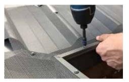
**STEP 8.** If standard or Mesh Lock trims are used, place the metal trim over the mesh at the gutter edge. The mesh should rest under the trim and against the front edge of the trim. Secure by placing a metal screw in every pre-made hole.
