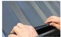
**STEP 1.** For 2mm mesh, pinch the mesh approximately 30mm back from the gutter edge to form a horizontal platform. This will create a water break to prevent water from flowing to the edge of the mesh during heavy rainfall. For 4mm or 5.4mm mesh, you should consider pinching the mesh when the roof pitch is steep (over approx, 30°)
