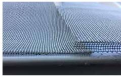
**STEP 4.** Before fitting the next sheet, notch the sheet out with tin snips on the formed edge so that it will allow the sheets to overlap each other by about 20mm. Fit as described in Steps 2-4.
