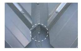
**CORNERS** Cut the mesh to the shape of the ridge capping. Overlap the mesh above the gutter and join using a metal screw.
