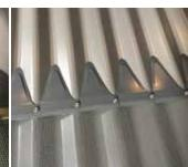
STEP 8. Screw to the roof sheet and continue along mesh length.
