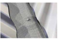
**STEP 4.** Secure each overlapping section of valley mesh together using metal screws provided. For narrower valley mesh, one screw per join is sufficient. For wider mesh, use two screws.
