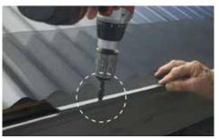
**STEP 3.** If standard or Mesh Lock trim is used, place the metal trim over the mesh. The mesh should rest under and against the front edge of the trim. Secure by placing a metal screw in every pre-made hole. Do not overtighten the metal screws.
