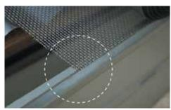
**STEP 1.** Place the roll of mesh on the roof with the cut edge of the mesh facing the gutter. The cut edge of the mesh should rest on top – and just inside – the edge of the gutter.
