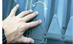
**STEP 2.** Place No.1 & No.2 multi-pitch fins over the mesh and on either side of the valley. Looking up the valley from the gutters internal corner, typically the No.1 multi-pitch fins are placed on the right and No.2 multi-pitch fins on the left.
