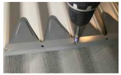
**STEP 6.** Move the Profile left and right to achieve a good fit. Screw to the roof sheet using the 3 middle screw holes.
