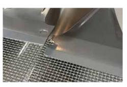
STEP 7. Overlap the profiles by placing the closed end screw hole over the open end screw hole. INSTALLATION TIP: Do not overtighten the metal screws. As a guide, tighten the screw to the point where the rubber washer begins to compress.
