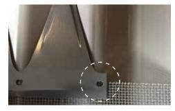
STEP 5. Place the profiles over the mesh.
