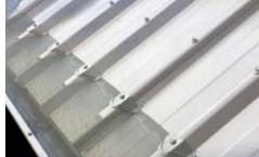
**STEP 5.** Place the saddle over the "U" shape and secure using a metal screw, then place a metal screw at the bottom of the "U" section through the mesh into the top of the rib. Do not over-tighten the metal screws. As a guide, tighten the screw to the point where the rubber washer begins to compress. For best results, use the mesh as a string line to keep the saddles straight.
