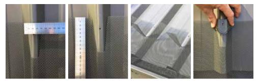
**STEP 4.** Secure the roof edge of the mesh by securing a saddle to every rib. Before installing the saddles, cut a "U" shape in the mesh about 40mm wide and 90mm long at every rib.
