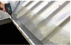
**STEP 3.** Place the standard or Mesh Lock trim over the mesh. The mesh should rest under and against the front edge of the trim. Secure by placing a metal screw in every pre-made hole. Do no over tighten the metal screws.
