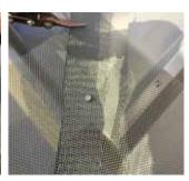
**CORNERS** Cut the mesh to the shape of the ridge capping. Overlap the mesh above the gutter and join using a metal screw.
