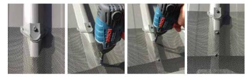
**JOINING MESH** When joining two pieces of mesh, overlap the mesh by 20mm. Place one metal screw through the centre of the overlap.
