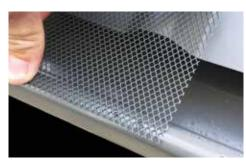
**STEP 1.** Place the roll of mesh on the roof with the edge of the mesh facing the gutter. The cut edge of the mesh should rest on top – and just inside – the edge of the gutter.
