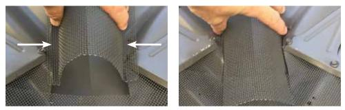
**STEP 2.** To fit the domed valley mesh, squeeze the mesh together until the folded edges fit beneath the roof sheet on both sides of the valley. Release the mesh so that it spreads and fits snugly under both edges of the roof.
