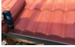
**STEP 2.** Roll the mesh out along the gutter edge. **INSTALLATION TIP:** Screw the mesh to the gutter at both ends to hold the mesh in place
