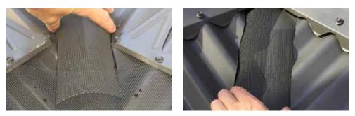
**STEP 4.** Start fitting the domed valley mesh at the bottom of the valley, 100mm up from the end of the roof sheet where it enters the gutter. Work up to the ridge overlapping each section by 4 mesh squares. The valley mesh should be fitted over the top of the regular gutter mesh at the bottom of the valley.
