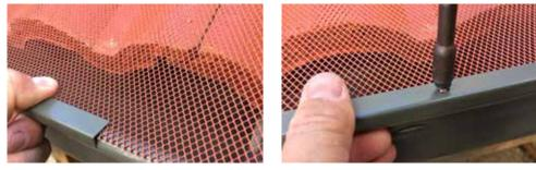
**STEP 3.** Place the standard or Mesh Lock trim over the mesh. The mesh should rest under and against the front edge of the trim. Secure by placing a metal screw in every pre-made hole. Do no over tighten the metal screws.
