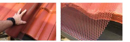
**STEP 1.** Place the roll of mesh on the roof with the edge of the mesh facing the gutter. The edge of the mesh should rest on top – and just inside – the edge of the gutter.
