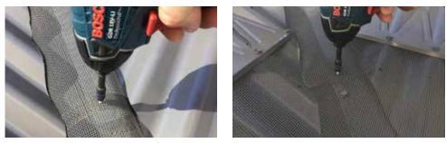
**STEP 5.** Secure each overlapping section of valley mesh together using metal screws provided. For narrower valley mesh, one screw per join is sufficient. For wider mesh, use two screws.
