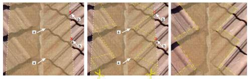
**STEP 3.** Using tin snips, cut the mesh on either side of the valley using points (a) and (b) as a guide. The notches (approximate thickness of the tile) created at point (a) will allow the mesh to transition from above to below the tile easily.
