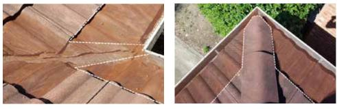
**CORNERS** Cut the mesh around the edge of the ridge capping. Overlap the mesh above the gutter and join using a metal screw.
