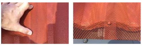
**JOINING MESH** When joining two pieces of mesh, overlap the mesh by 20mm. Place a metal screw through the centre of the overlap.
