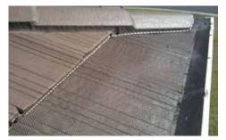
**STEP 6.** If the hips and gable ends are secure with concrete, you will be unable to lift the second tile. Instead, cut the mesh to be in line with the front of the second row of tiles and seal with silicone (if required).
