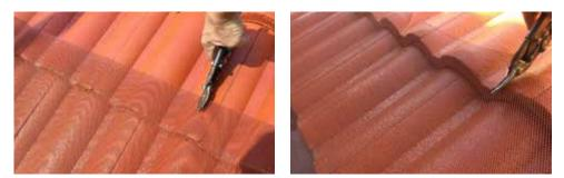
STEP 4. Using offset tin snips, cut a slit in the back of the mesh next to the overlap in every tile.
