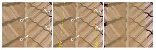
**STEP 2.** Determine two points up the valley where the mesh will transition from over the tile to under the tile (a), and length of the flap which will be tucked under the tile (b), all the way up the valley on each side. Using tin snips trim the excess mesh away where these two points intersect up the valley on each side.
