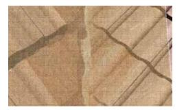
VALLEYS (ALUMINIUM MESH)STEP 1. Roll out the required length of gutter mesh along the valley gutter.NOTE: Valley mesh should be installed last to ensure it sits on top of the gutter mesh previously installed at the gutter.
