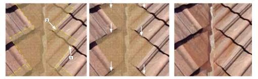
**STEP 4.** Using a flat head screw driver, lever the upper tile off the lower tile (1) and then tuck each flap created previously (2) under, before lowering the tile back in place. Press down firmly to lock the mesh into position being careful not to damage the tile.
