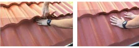
**STEP 5.** Tuck the mesh under the tile by lifting the second row of tiles from under the mesh. Use a flat head screwdriver to lever the second tile up as required.
