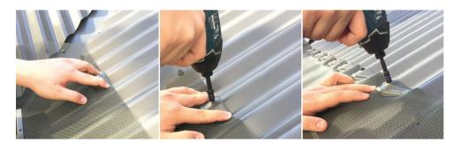
**STEP 6.** Place the saddle over the flap/tag and secure using a metal screw. Do not over tighten the metal screws.
