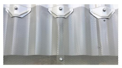
**JOINING MESH** When joining two pieces of mesh, overlap the mesh by 20mm. Once it's in place, insert a metal screw through the centre of the overlap. Fasten until the overlap pulls together.
