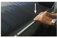
**STEP 4.** For 2mm mesh, pinch the mesh at the gutter edge to form a horizontal platform. This will create a water break to prevent water from flowing to the edge of the mesh during heavy rainfall. For 4mm or 5.4mm mesh, you should consider pinching the mesh when the roof pitch is steep (over approx, 30°).
