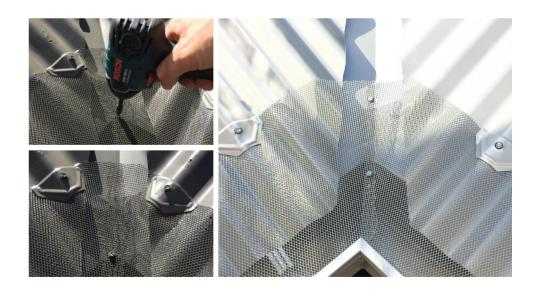
**CORNERS** Cut the mesh to the shape of the ridge capping. Overlap the mesh above the gutter and join using a metal screw.
