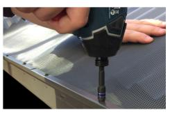
**STEP 3.** Place the standard or Mesh Lock trim over the mesh. The mesh should rest under and against the front edge of the trim. Secure by placing a metal screw in every pre-made hole. Do not over tighten the metal screws.
