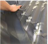
**STEP 2.** Cut two slits about 20mm apart and 30mm long at the same angle as the corrugation to create a flap/tag at every rib on both sides of the valley.
