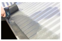
STEP 2. Roll the mesh out along the gutter edge.
